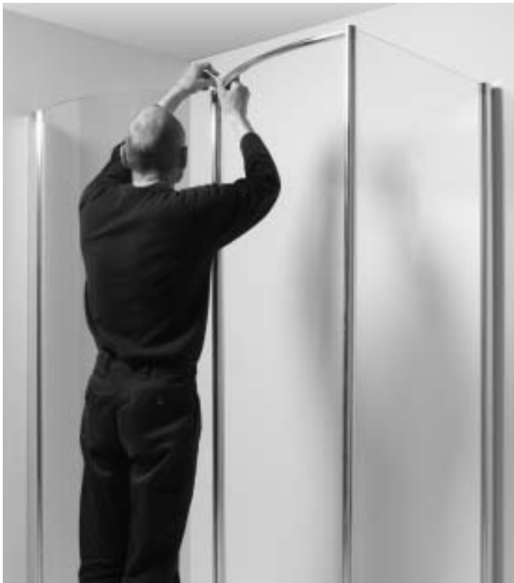
7 Place longer support rail V1151 from side panel to main panel into position.
