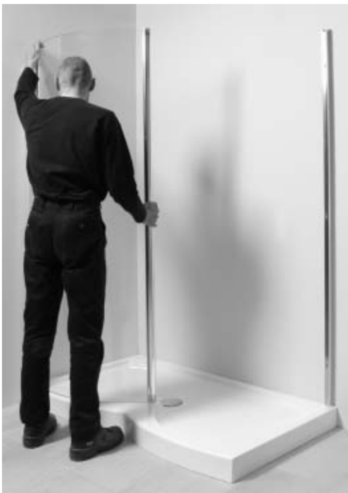
5 Place main glass panel A into position and drill holes in the upright profile, as shown at 6, into the wall profile and secure with screws V4150, clips V2151, and cover caps V2151.
