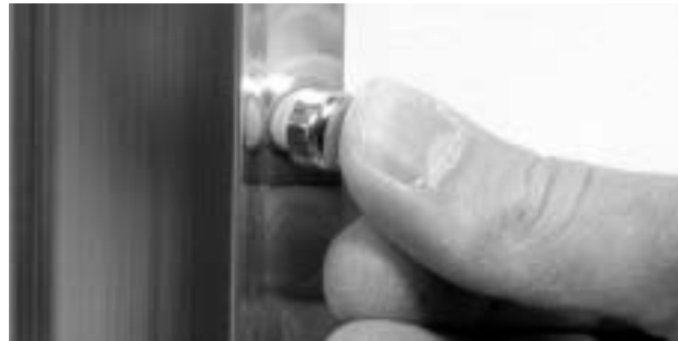
5 Place main glass panel A into position and drill holes in the upright profile, as shown at 6, into the wall profile and secure with screws V4150, clips V2151, and cover caps V2151.
