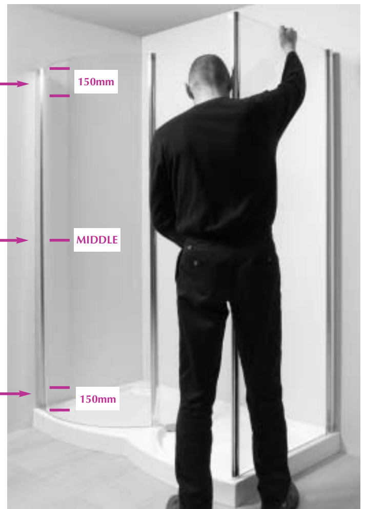
6 Place end glass panel B into position and fix as shown at 5.
