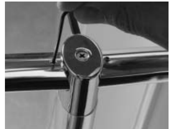
9 Secure rail mounting bracket to wall. Re-fit rail and tighten all retaining grub screws in rails.
