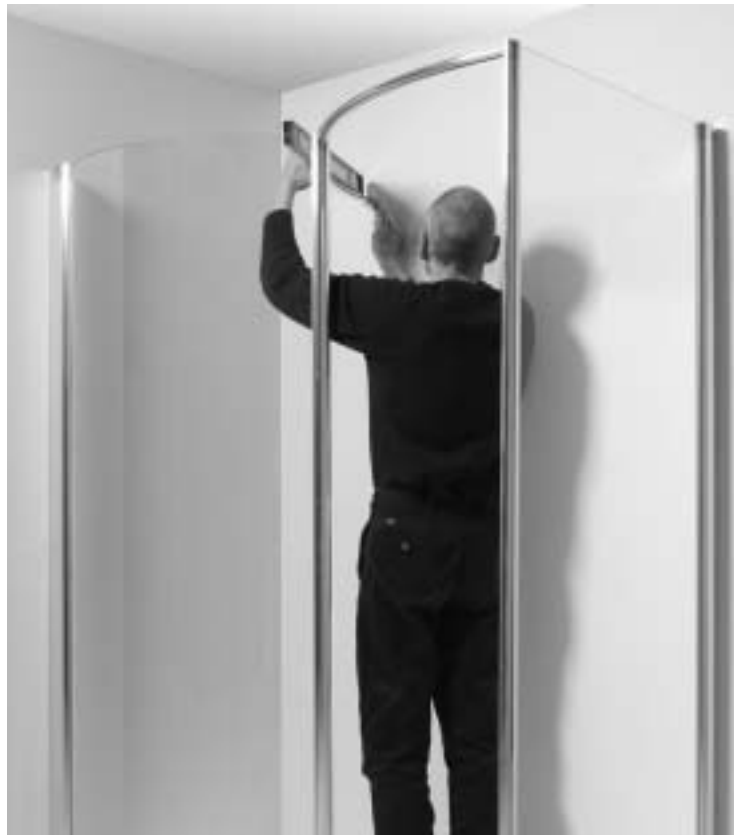
8 Place shorter, main panel support rail V1152 into position, level and mark position for mounting bracket.
