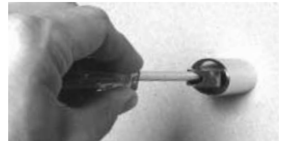
Picture shows fixing for installation with main panel and end panel. When installing main panel only turn bracket through 90° to fit rail V1153.
