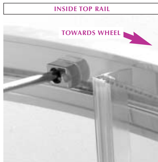
14 Fit SHORT roller stop V6104 into the pre drilled hole on the inside of the top profile. Insert cover caps V2111 to all roller stops.
