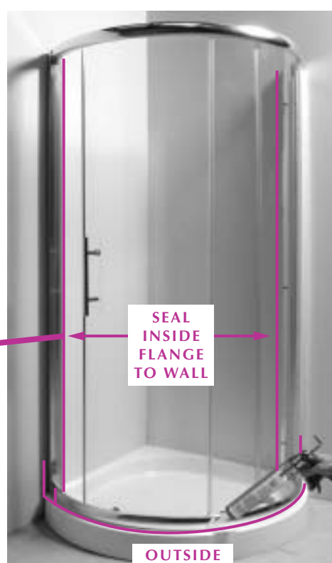
17 When doors are operating correctly & magnetic seal is fully aligned proceed to sealing of unit.
