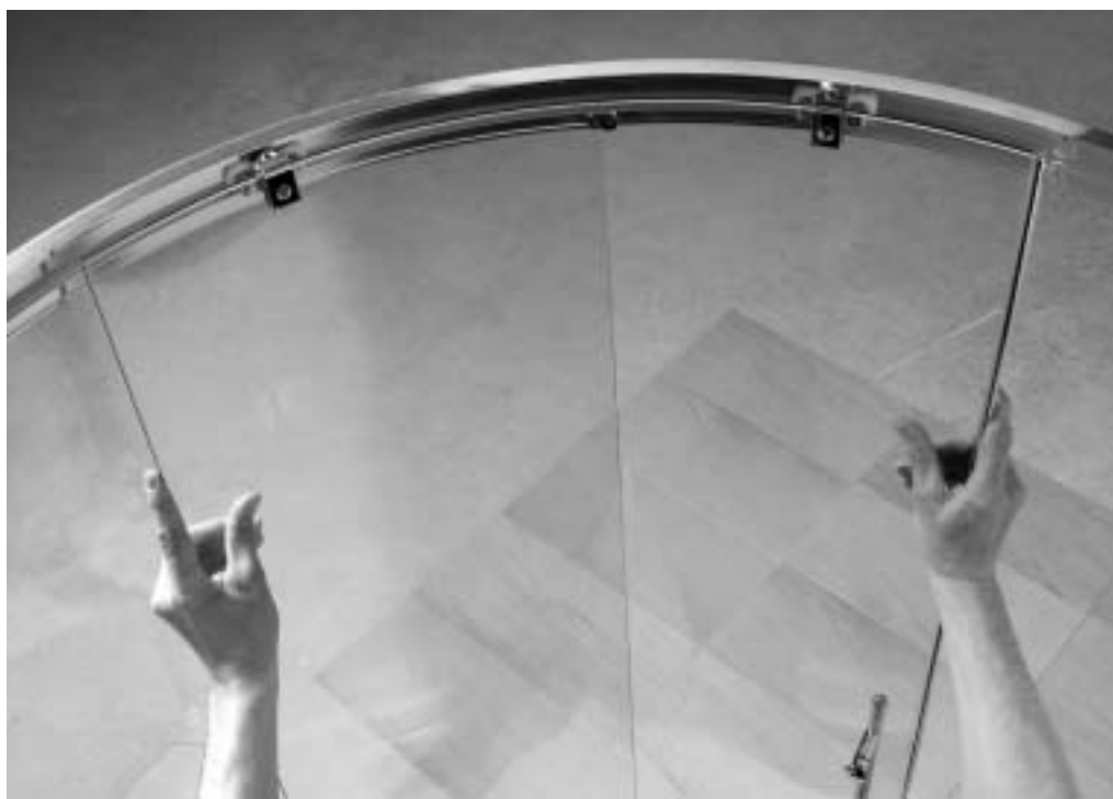
10 Working from inside the enclosure. Fit door onto top rail. Double rollers on top
