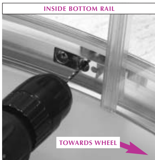
13 Screw the back hole of the LONG roller stop V6105 to the pre-drilled hole on the inside of the bottom profile. Drill through the front hole and screw. Insert cover caps V2111.
